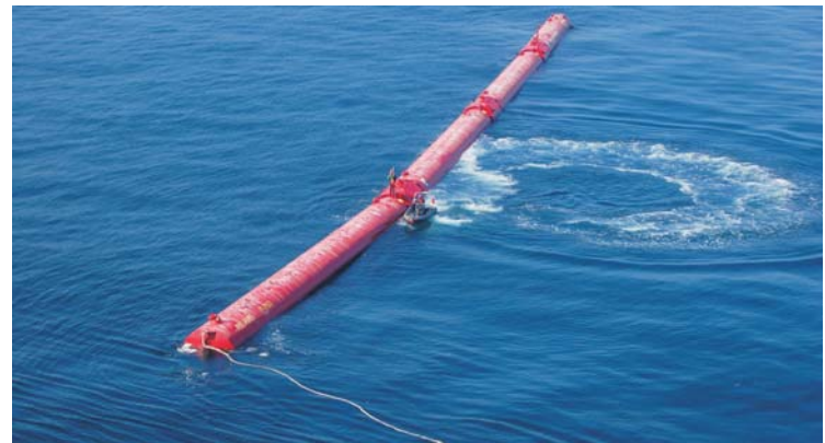
Wave-energy power plant.
